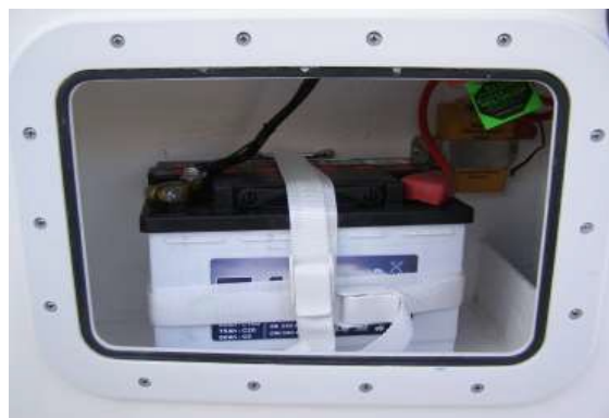
Opened hatch w/battery
